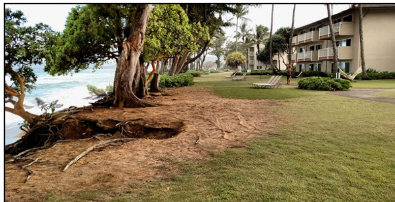
Erosion at Kaua'i Coast Resort at the Beachboy
